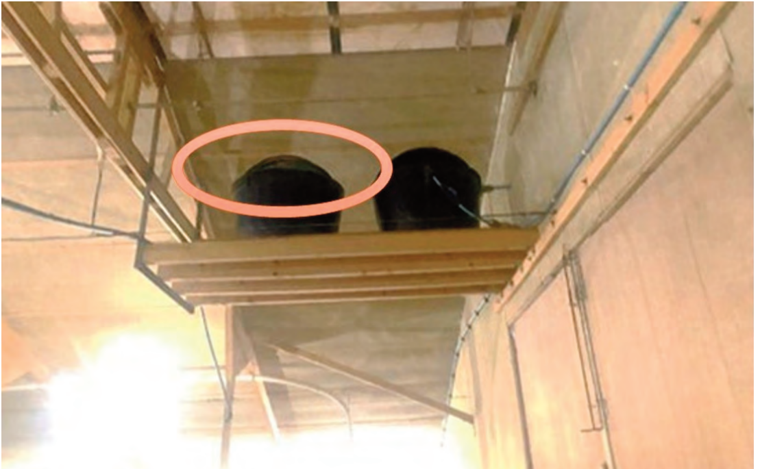
Poor - water header tank lid appears to be incompletely secured potentially allowing access by rodents.
