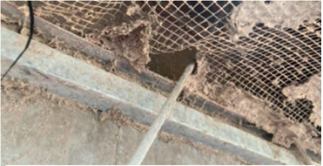
Poor - gaps in meshing covering ventilation inlets.
